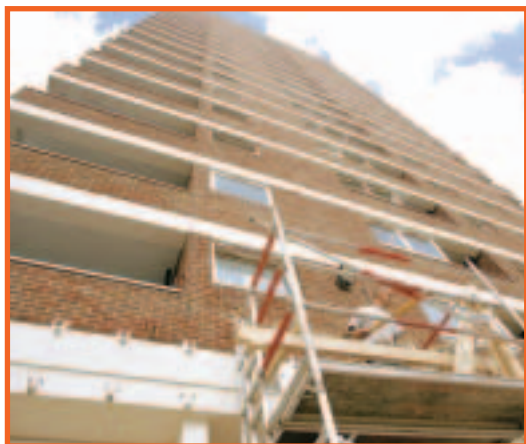
Sustainable refurbishment taking place on Integer's Westminster Towers project.
